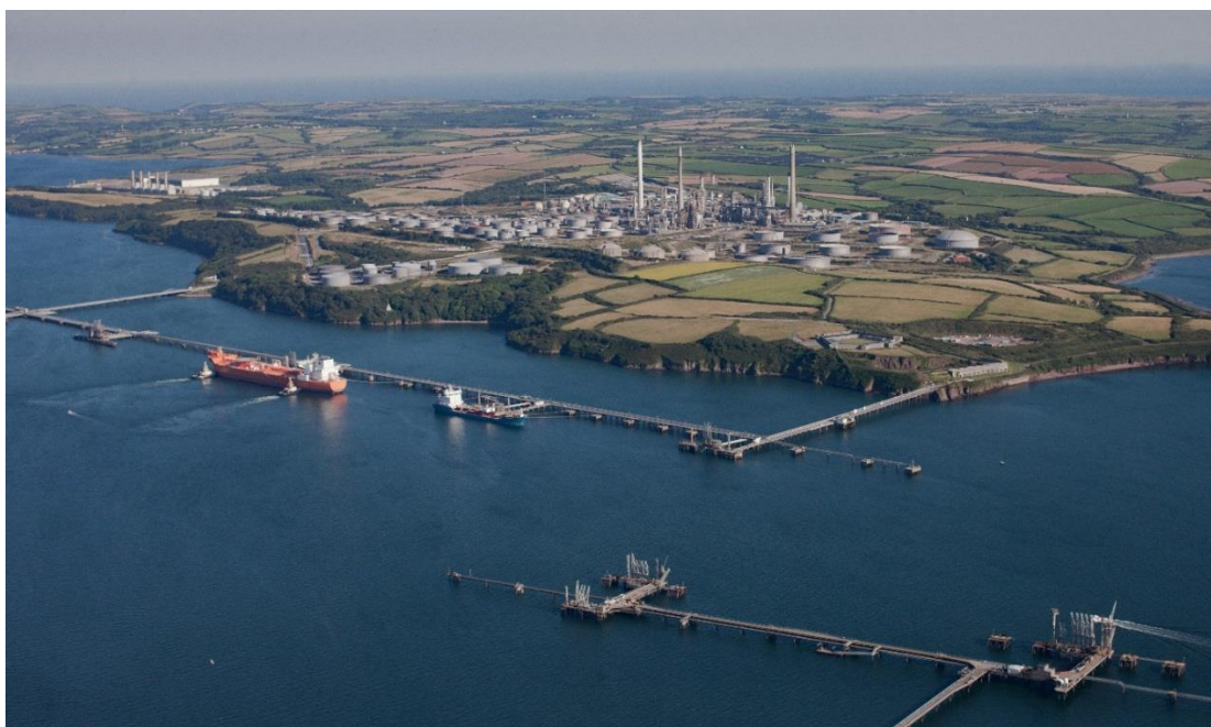
Pictured: Pembroke Refinery
